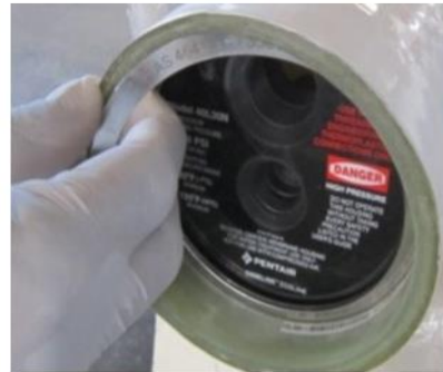
Removal of Retaining Ring
