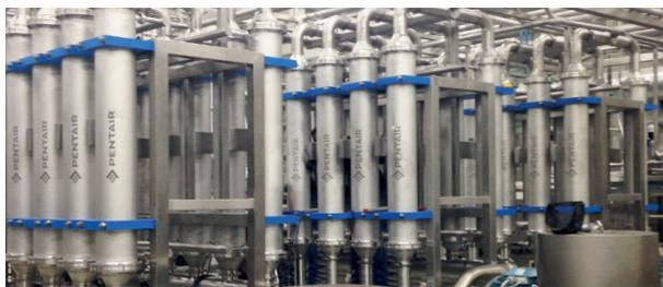
Four membrane units - Capacity to treat 6 ton/h of skimmed milk
