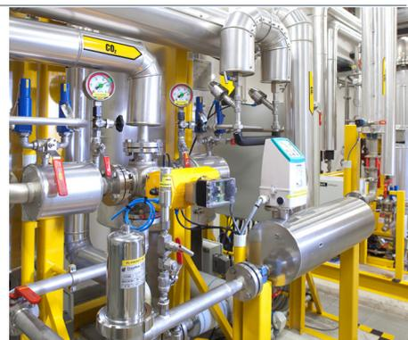
Flow Meter mounted on skid with Activated Carbon Filters/Dryer
