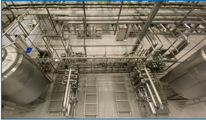
Top view on Pentair Beer Membrane Filtration System at Hanuman
