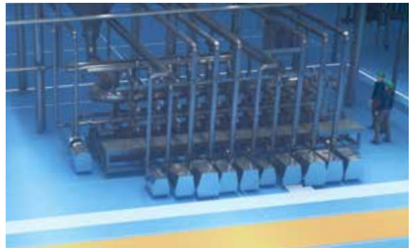
Deaerated Water Distribution
